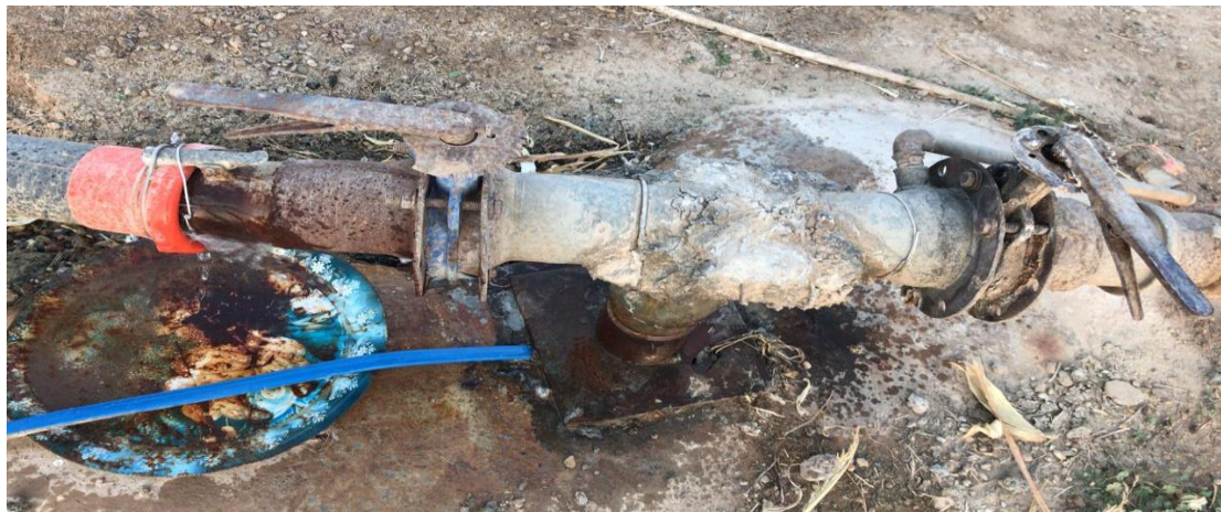
Figure 3. Well No. (6) Jalam Al-Dur
